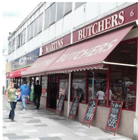
This shop has a well-designed fascia and canopy
