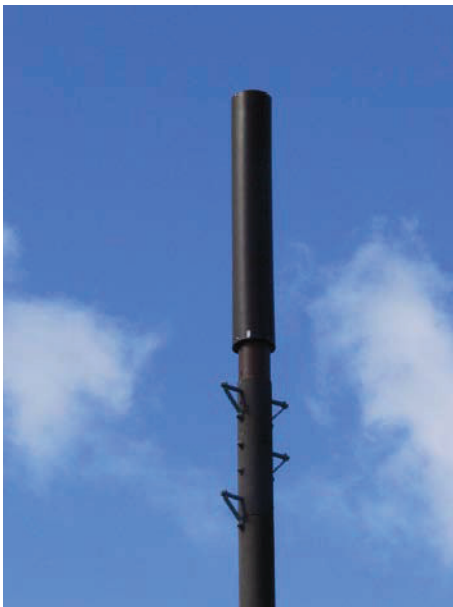
Examples of camouflaged telecommunications equipment
